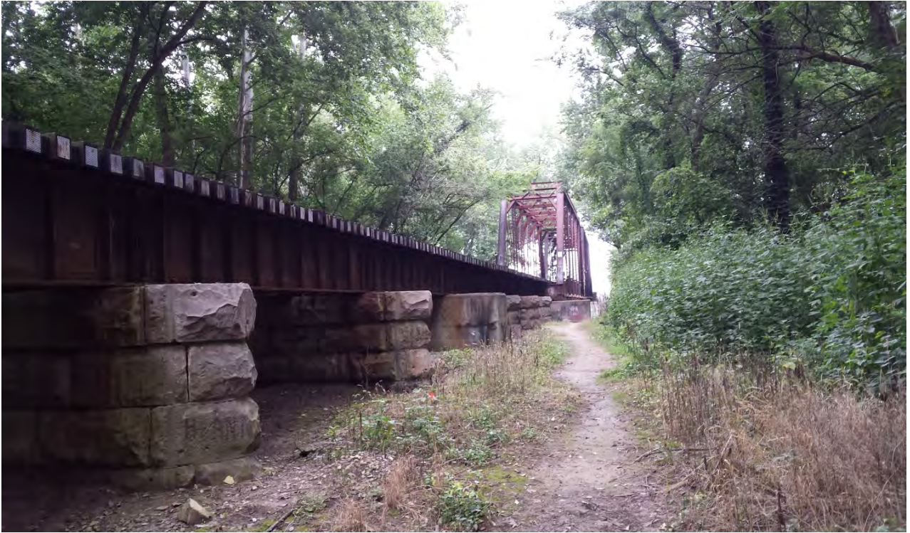
Photo 1. Flatrock River bridge and spans looking north
